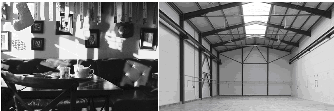
Fig. 1: Influence of direct daylight on building interior: left – visual discomfort in the side lit interior; right – visual comfort in an industrial hall with the diffusive roof skylight
